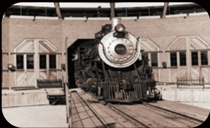
Engineer Al Shelley moves Santa Fe No. 1010 out of the Museum roundhouse.
